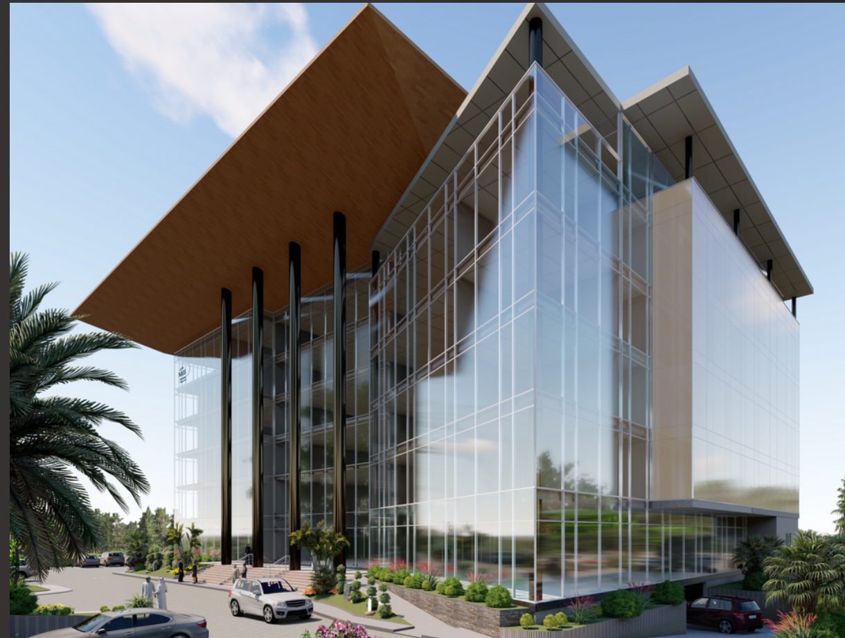
NASS HEADQUARTER AT SALMABAD
